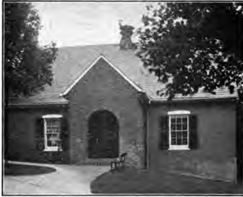
The Old Treasury Building, Annapolis 1
